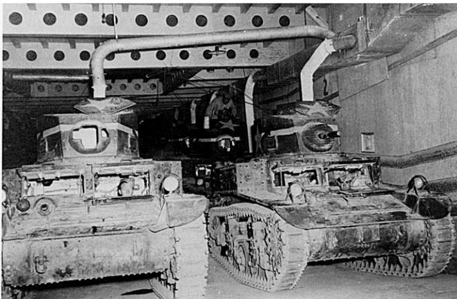
After a few tanks had been parked inside the LST Building, large flexible ducts were attached to each tank's engine exhaust in order to disperse their noxious fumes to the atmosphere, as shown on the left.
