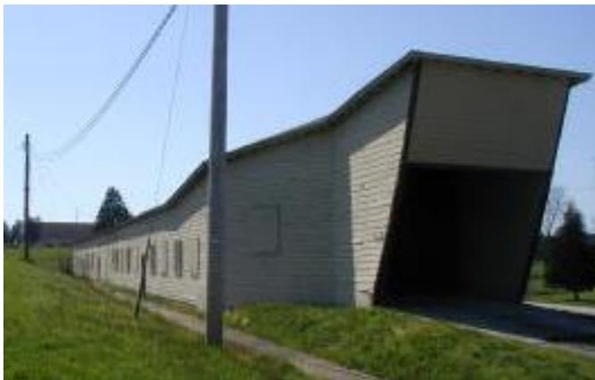
After lying dormant for about three years, the all wooden structure was converted into classrooms. Windows and doors were cut into the sides of the structure. Heating and fire protection systems, and restrooms were installed. For three decades the US Army's Armor School used the building for educational purposes.
