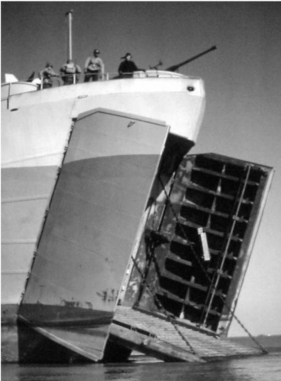
'Clam shell' doors and a ramp were fitted to their bows. Machinery and crew spaces were mostly located aft, allowing for as many as 27, twenty-five ton tanks to be carried internally.
