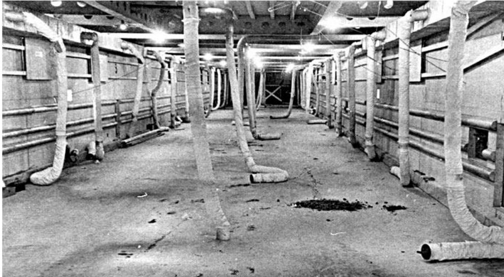
Bureau of Ships observers decided that a better design was needed. The ultimate fix was to install several huge fans in the overhead of the tank deck of all LST's. These fans discharged directly to the atmosphere, keeping the enclosed area reasonably clear of noxious fumes. After this concept was tried in the 'Fort Knox Ark' and found acceptable, all testing there ended in August of 1942.
