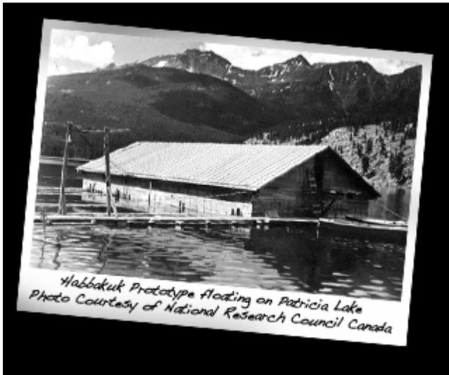
When the structure, topped with a roof to protect the refrigeration equipment was freed by that year's spring thaw, it floated as expected. In June of 1943, the refrigeration equipment was switched off. But the ice-ship prototype took all summer to melt before allowing the prototype's cooling equipment to sink to the bottom of the lake. Where it still remains, greatly deteriorated, but marked by a suitable plaque placed underwater that serves today as a curiosity for recreational divers.
