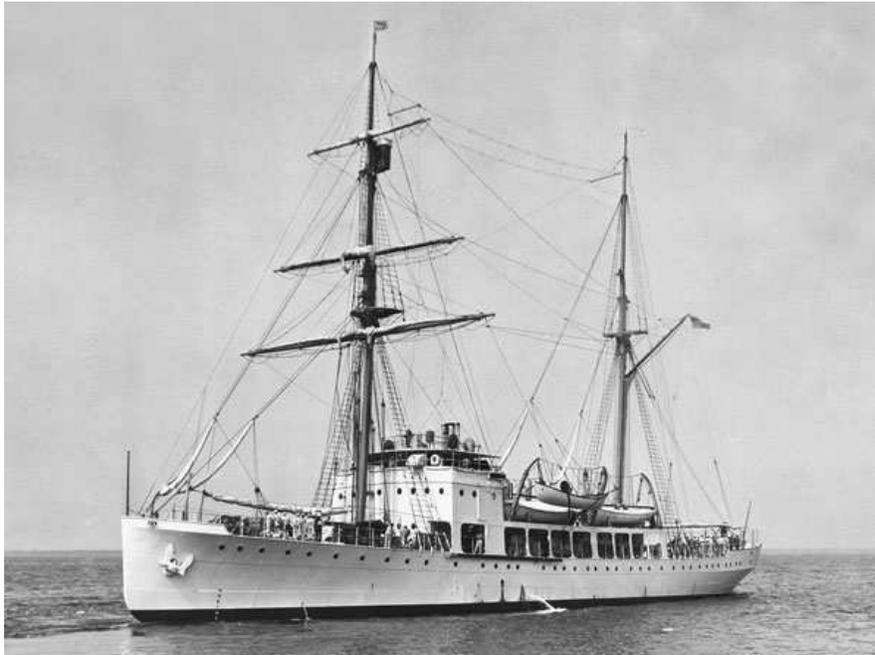
Before the NORTHLAND was designed, wooden and even riveted steel hulls of Coast Guard cutters that served in Arctic waters were often compromised by the unremitting pressures of sea ice. Under adverse conditions, hull seams were opened up at times, causing flooding. Occasionally, relatively fragile hulls were even crushed. To overcome that problem, in 1926, the Coast Guard specified the extensive use of welding in the construction of NORTHLAND.
